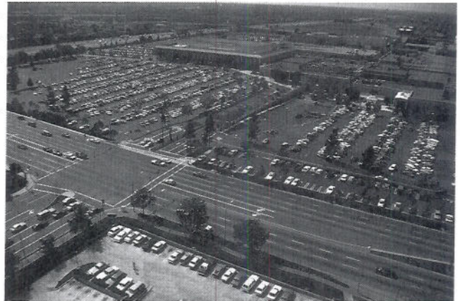
Suburban development often demands extensive amounts of land for parking and multi-lane two-way streets.
