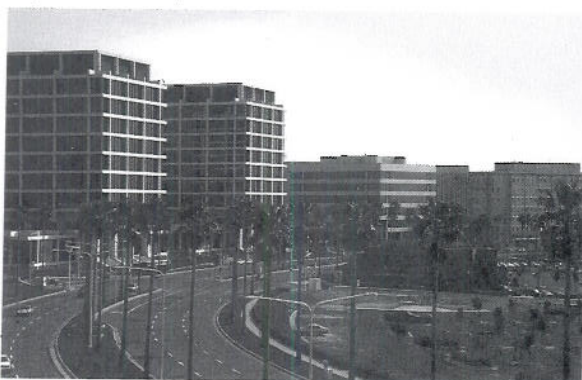
High-rise office development moves into the suburban fringe where land is cheaper and auto access is easier.
