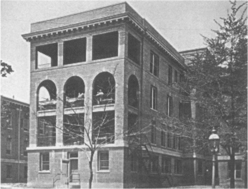
Figure 5: Porches, Children's Hospital of the District of Columbia, 1928. Porches not only reinforced the domestic nature of the hospital, they also served as spaces for fresh air treatments and viewing places for parents to see their children. Source: Edward F. Stevens, The American Hospital , 3rd ed., 1928, in the author's collection.
